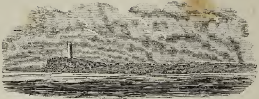
View of Montauk Point, Long Island.
